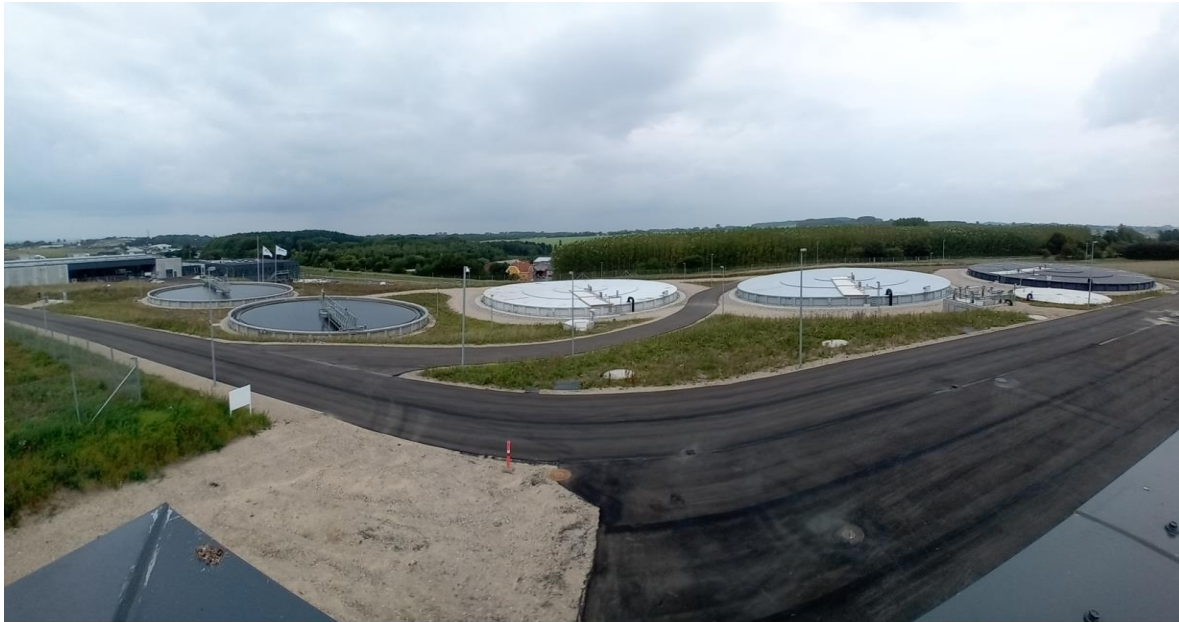
Panorama from roof of inlet works. Primary settlement to the right, two large aeration tanks in centre with smaller brewery specific tank to the right, two final settlement tanks to the left and office plus and workshop buildings to the left
